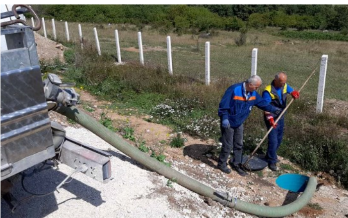
CONSTRUCTION AND MAINTENANCE WORKS AT NEW SITE LIPA © IOM 2021 © IOM 2021
